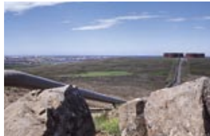
Hot water storage tanks at Grafarholt near Reykjavík.
