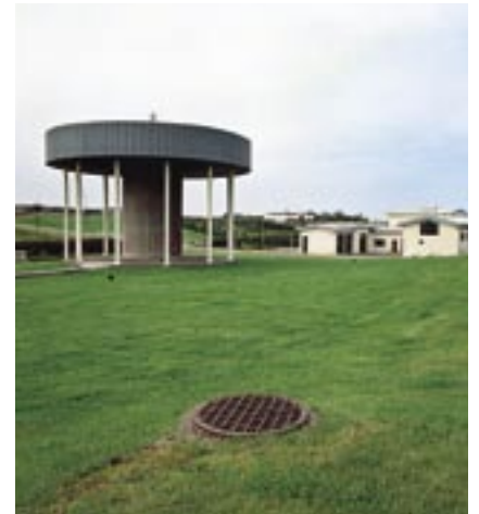
Pumpingstation at Reykir Mosfellsbær.
