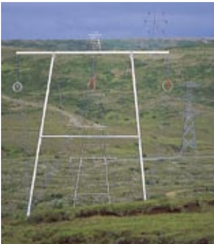
The transmission line.
