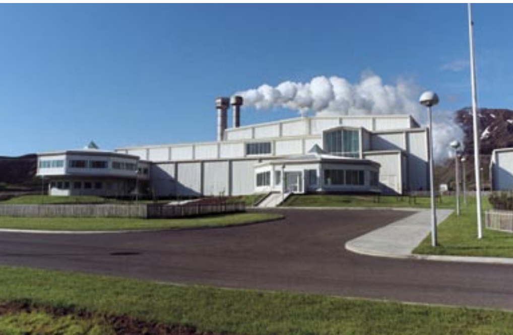
The power plant at Nesjavellir.
