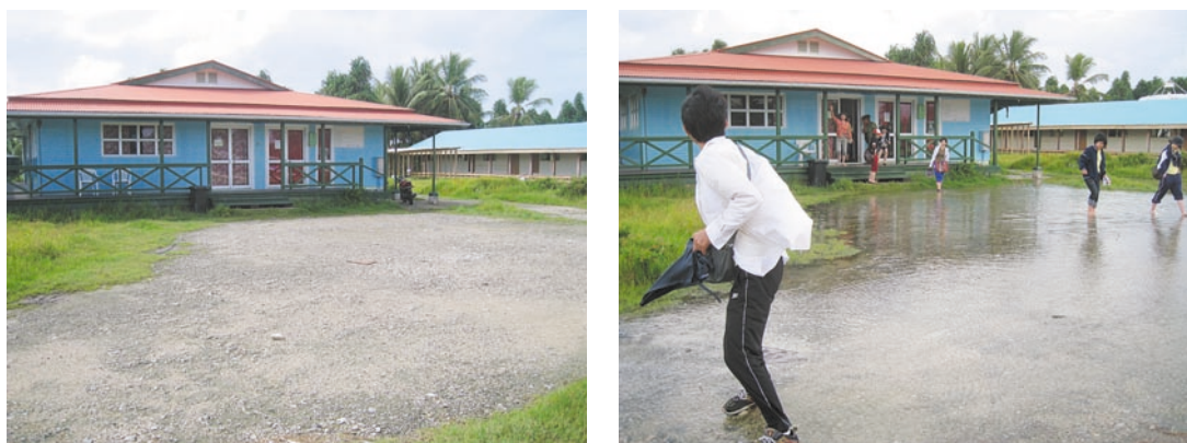
(Fig. 12-1, 12-2 Inland flooding in front of TUFHA)
