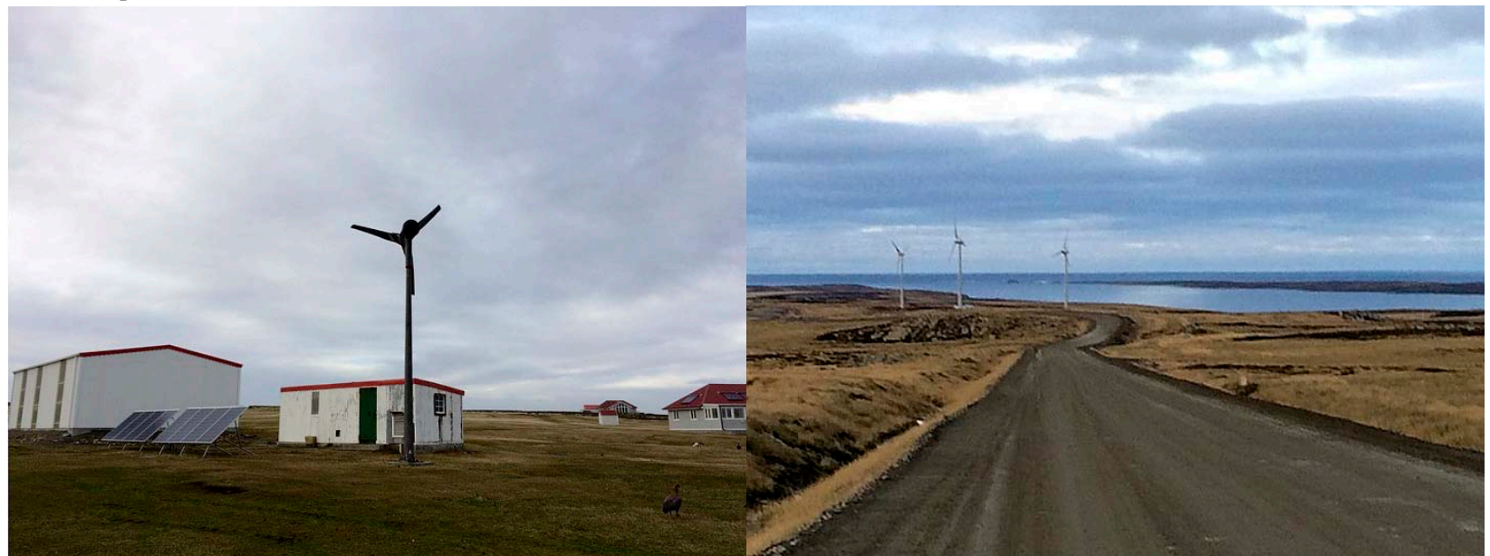
Small- and larger-scale wind-power generators in the Falkland Islands (Falkland Islands Government)
