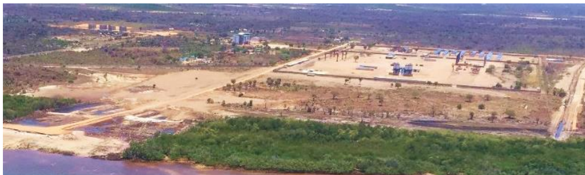
Figure 10: Port of Lamu – Construction Phase
